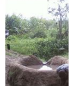
Emping of water trough immediately after construction (Tanzania)
